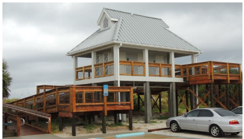
Figure 1: Elevated public restroom with extensive ramp that obstructs wave action, and is nearly twice the footprint of the base building.
